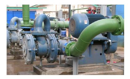
TEFSA can provide high quality for high solid's pumps sludges concentration and products. The main types (but not limited to) are centrifugal and pneumatic pumps:
