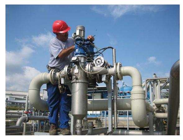
Self cleaning filters are easy to place and install. They can be placed in any section of horizontal pipe with liquid impulsion.
